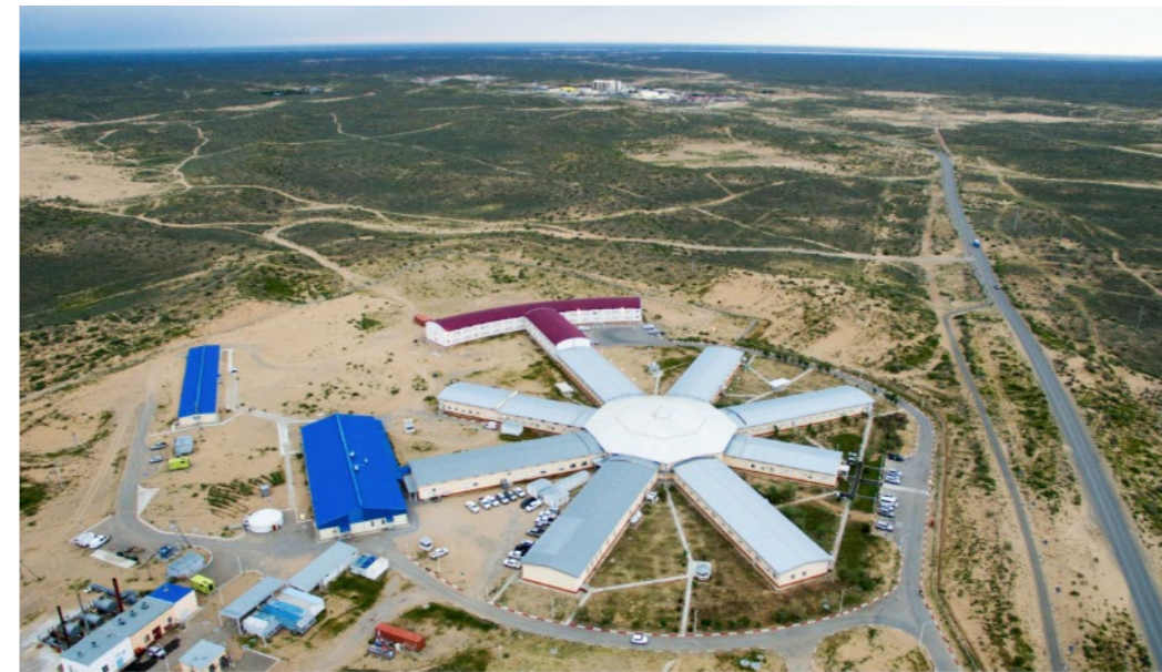
Uranium production in Kazakhstan (Source: Kazatomprom)
